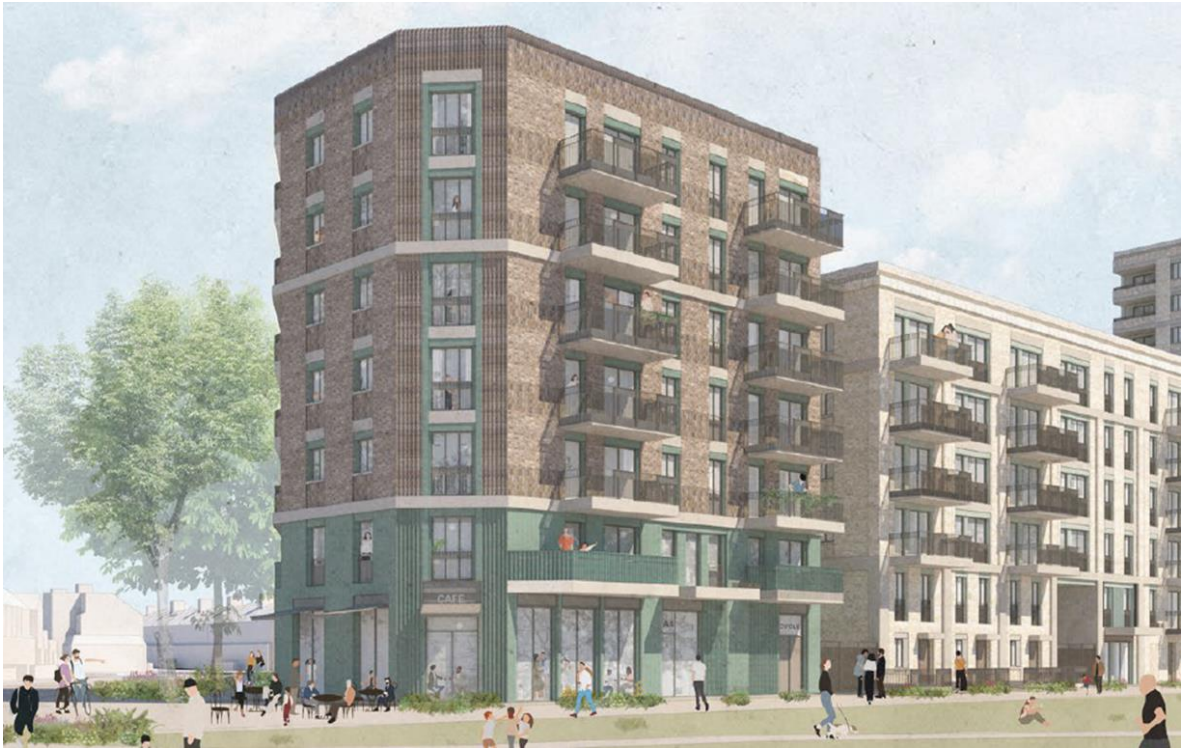
Image of Council homes currently being built at Ashley Road development – view from Park View Road (West)
